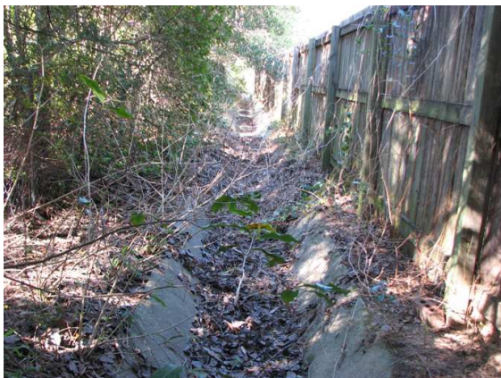
Drain areas located behind 1224 and 1228 are clogged with leaves and sand. Some shrubs and other growth also need to be cut back.
