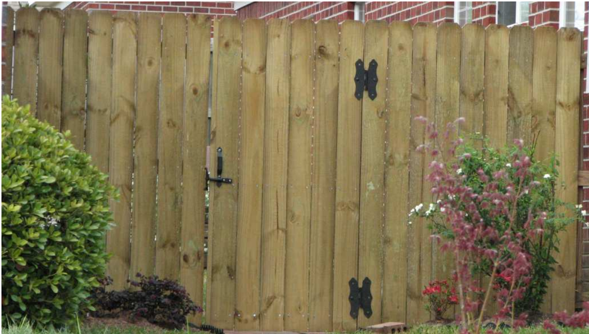
Front portion of fence built by Charles Snyder between the Snyder and Shumacher homes
